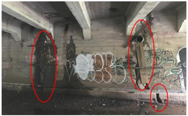
Image 7: Large Cracks in Right Bank Wall and Foundation
