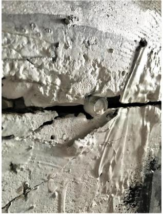
Image 19: Failed Crack Injection
