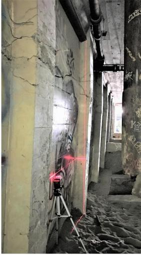
Image 14: Self-leveling Laser at Interior Pilaster
