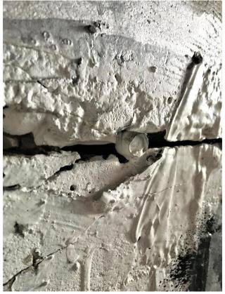
Image 21: Failed Crack Injection
