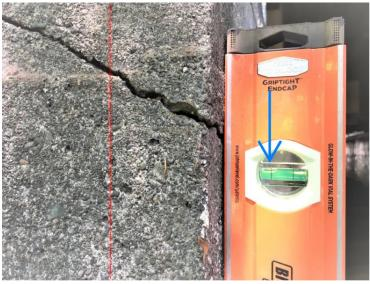
Image 11: Southern-most Pilaster w/ Level Bubble
