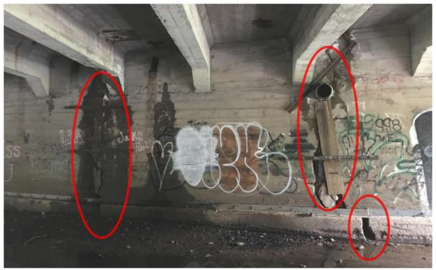
Image 5: Large Cracks in Right Bank Wall and Foundation
