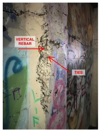
Image 14: Exposed Rebar at Pilaster
