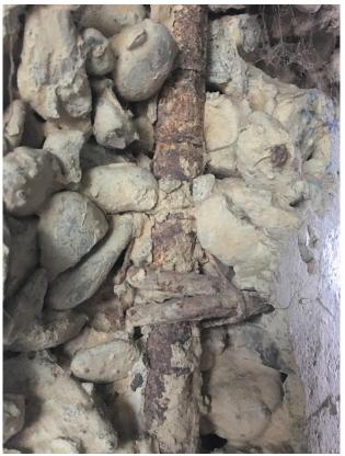
Image 17: Exposed Rebar Close-up
