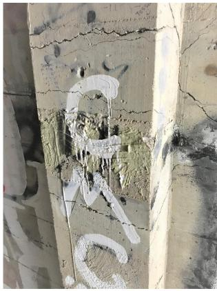
Image 20: Signs of Previous Crack Repair
