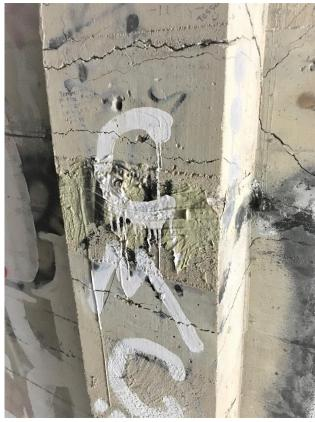
Image 18: Signs of Previous Crack Repair
