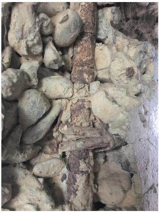
Image 15: Exposed Rebar Close-up
