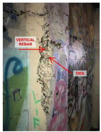
Image 16: Exposed Rebar at Pilaster
