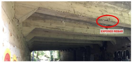
Image 4: Beam Deterioration at Bottom Face and Expose Rebar
