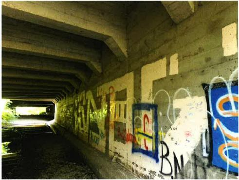
Inside face of structure is near original condition and structurally sound.
