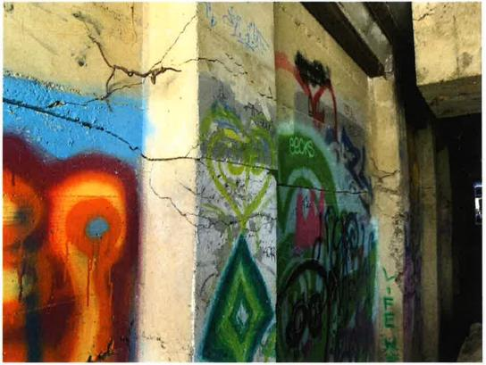
Cracking due to tension on the back face of the Pilasters/Columns
