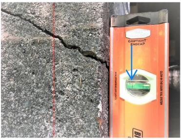
Image 13: Southern-most Pilaster w/ Level Bubble
