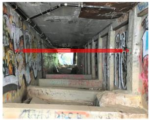
Image 26: Schematic of Temporary Horizontal Shoring (one location shown)
