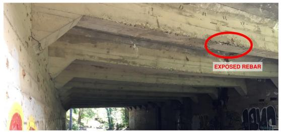
Image 6: Beam Deterioration at Bottom Face and Expose Rebar
